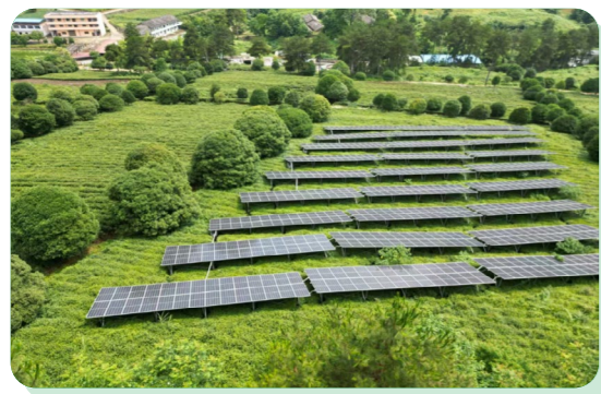
The Beipiao Photovoltaic Power Plant in Liaoning Province realized comprehensive land use through "power generation on panels, cultivation between panels and grazing beneath panels"
