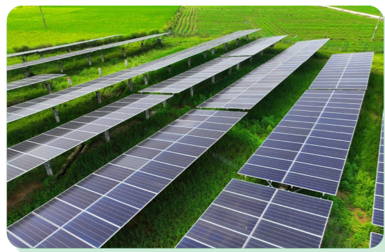
The "aquavoltaics" project at Bihu Fishery in Hunan Province generated photovoltaic power on the upper layer and conducted aquaculture on the lower layer, bringing benefits to fishermen and economic gains to the local government
