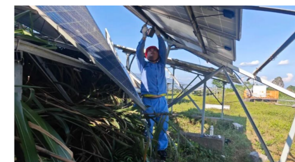
Conduct emergency repairs after typhoons
